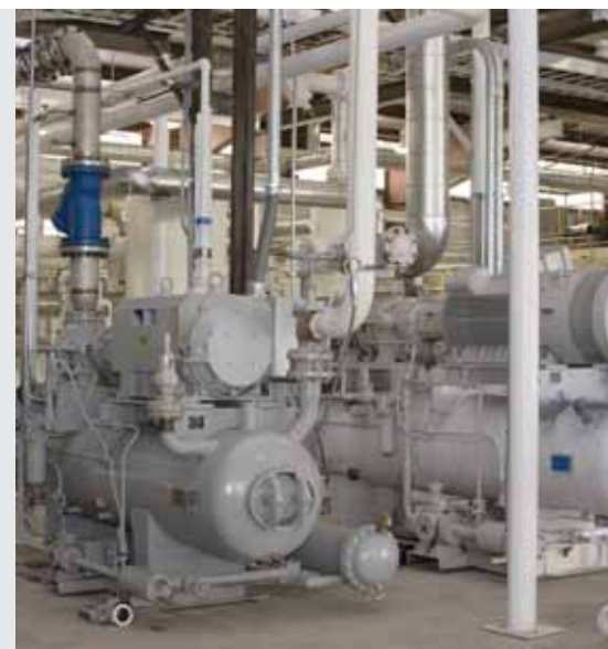
Speed Control of lead Compressor plus one more, offers improved and streamlined design possibilities and a better choice of Compressors sizing to adapt to varying load conditions
